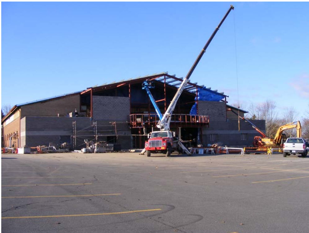
Current Renovations to the Amherst Stadium
