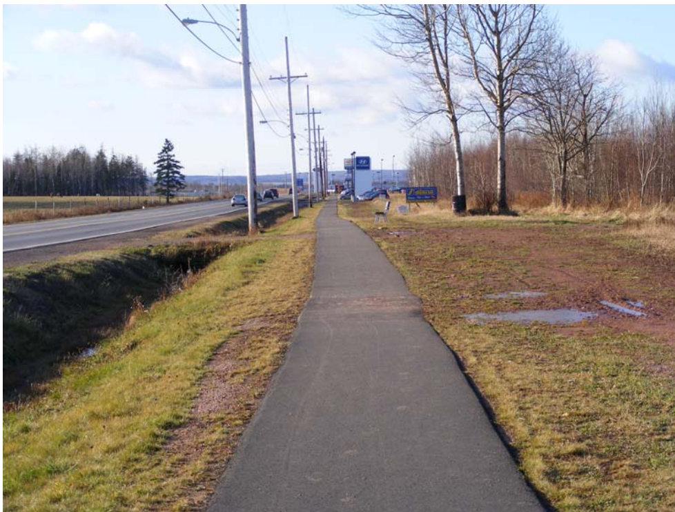
New Sidewalk in Developing Commercial Area
