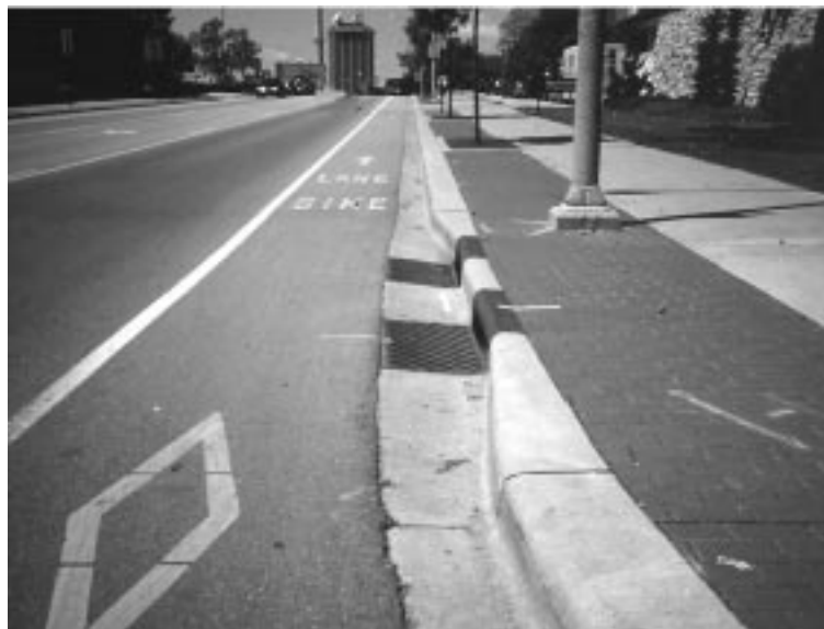
Urban drainage. RATING: Excellent
