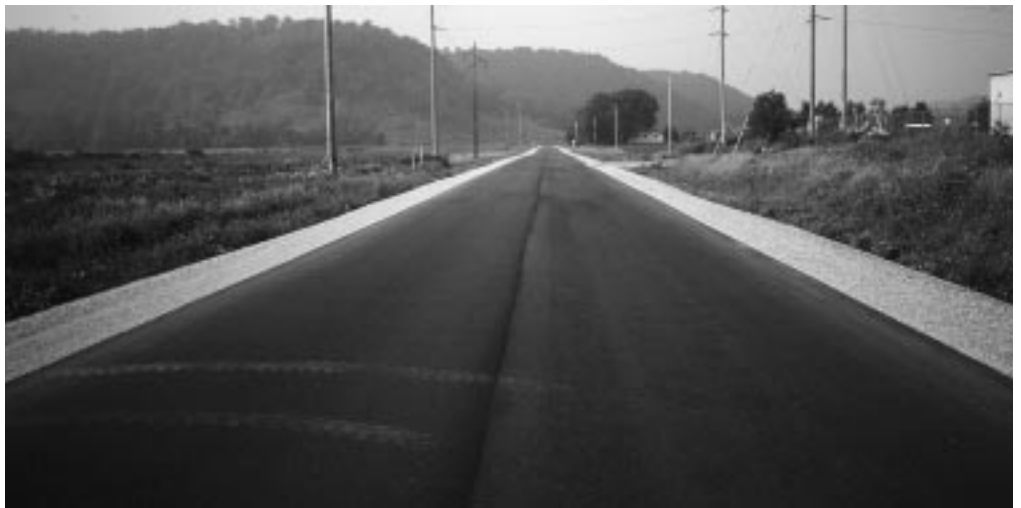
▶ RATING 9 Recent overlay, rural.
