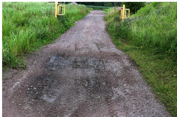
TIRE TRACKS FROM ATVs ARE WORN INTO THIS SECTION OF THE TOWN OF AMHERST'S MARSH TRAIL. TOWN OFFICIALS ARE RESPECTFULLY ASKING ATV OPERATORS TO REFRAIN FROM USING THE WALKING AND CYCLING TRAIL. (TOM McCOAG / TOWN OF AMHERST)
