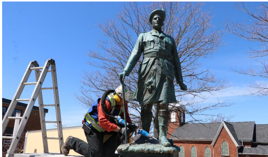
ED BOWKETT OF HERITAGE GRADE ARCHITECTURAL RESTORATION SERVICE BEGINS ICE BLASTING THE SCULPTURE THAT IS THE FOCAL POINT OF THE CENOTAPH IN AMHERST. (TOIM McCOAG / TOWN OF AMHERST)
